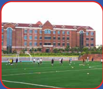
HARROW INTERNATIONAL SCHOOL, DEVANAHALLI
